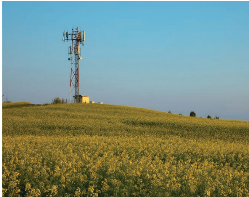
The project consists of MNOs investing to extend their coverage by upgrading their existing networks, working together on shared infrastructure and building new sites, with new government-funded masts being built to target areas with no mobile coverage from any operator
