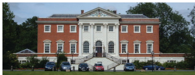
The DXC team transitioned the council’s network from Juniper SAs to Pulse PSAs in a two-day, on-site implementation project “with minimal interruption” to services
